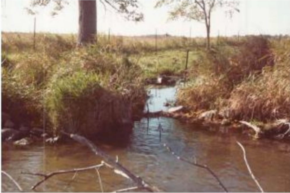
Figure 1 1983 Photograph of the Loose Rock Dam on Somers Lake (photo courtesy of the MNDNR)
